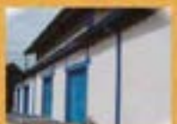
Warehouse Complex Mount Lavinia
